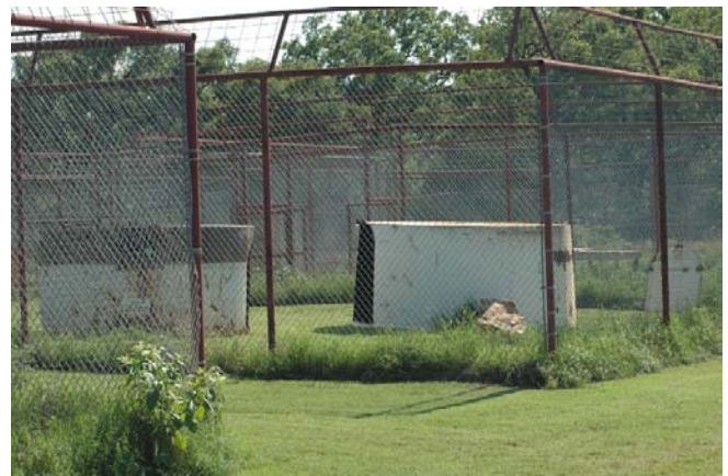
This picture shows a habitat that is currently under construction in the lower compound at CARE's facility.
